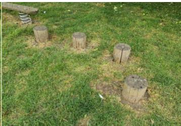
**Finding:** There are areas or parts of the timber posts on the **Action:** Replace all affected timbers structure that have rotted
